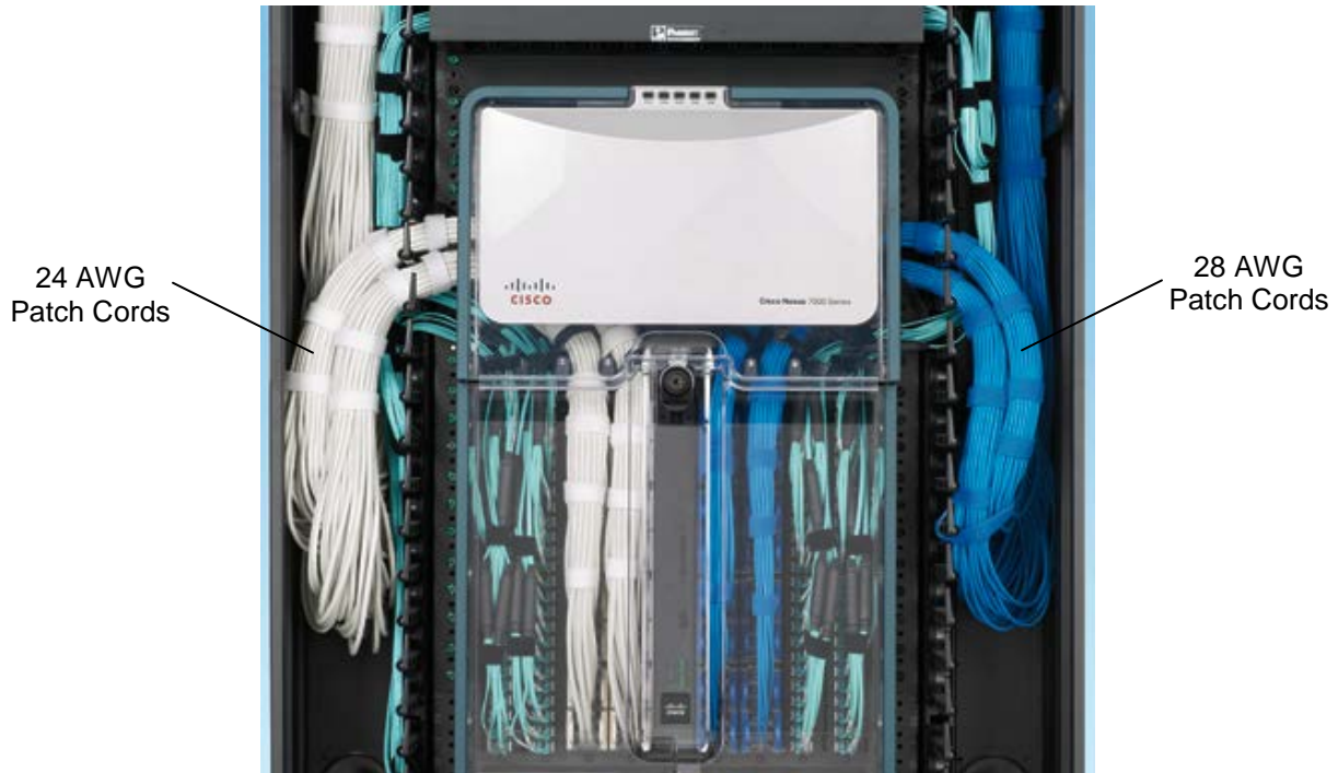
Figure 1 – 24 AWG Patch cords (white) vs. 28 AWG patch cords (blue)
